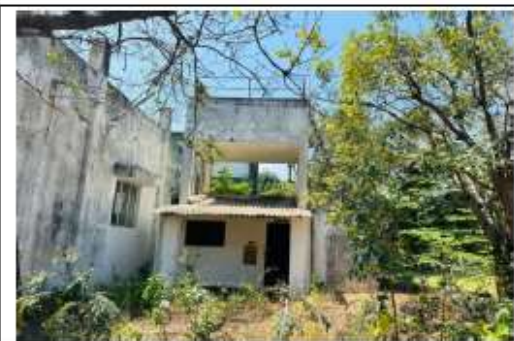
OHT AREA VIEW
