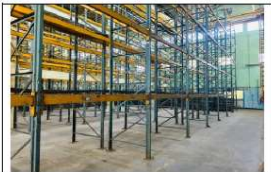
STORAGE GODOWN VIEW
