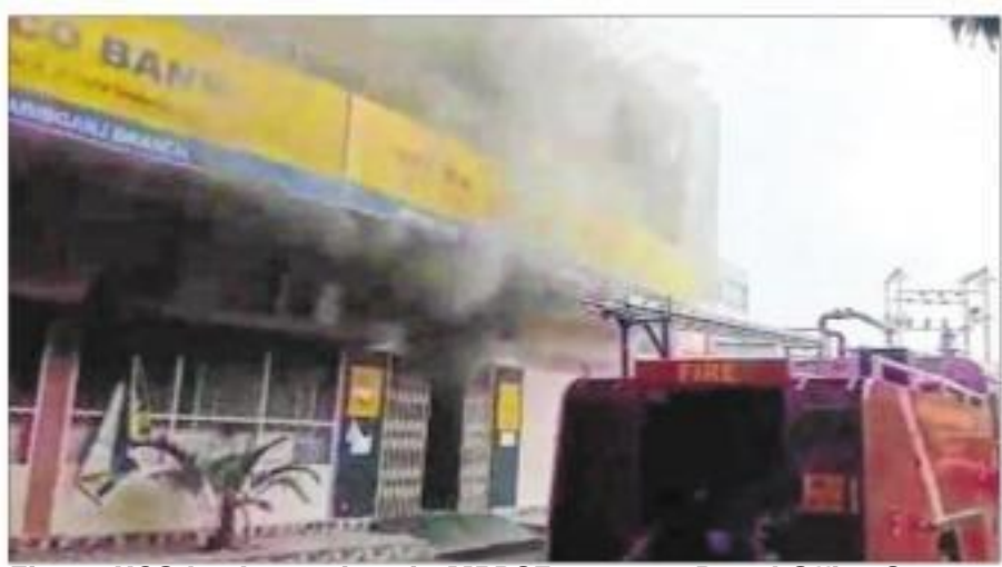
Fire at UCO bank premises in MPBSE campus, Board Office Square
